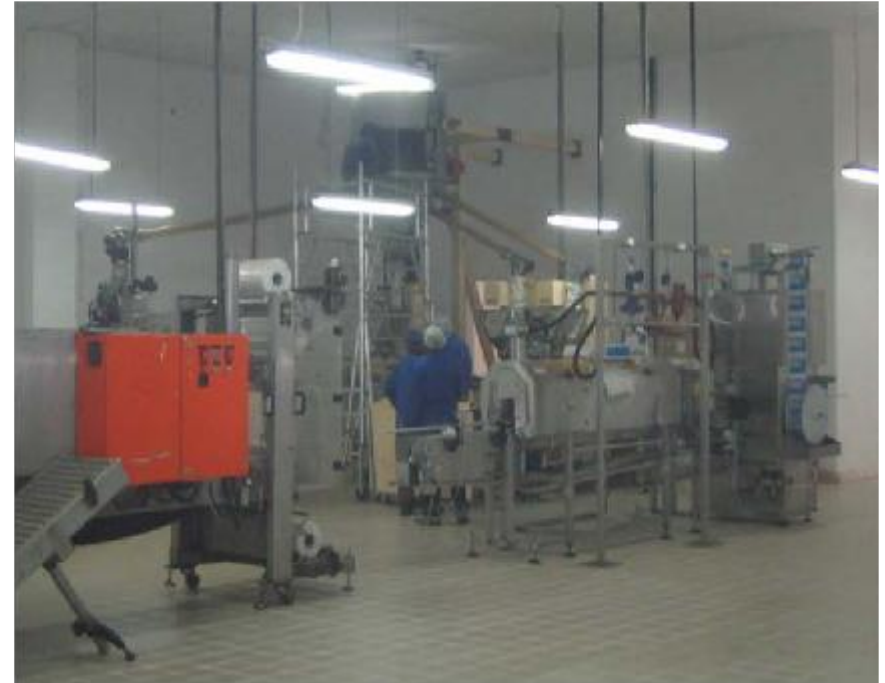
Facility upgrade – new sleeving line
